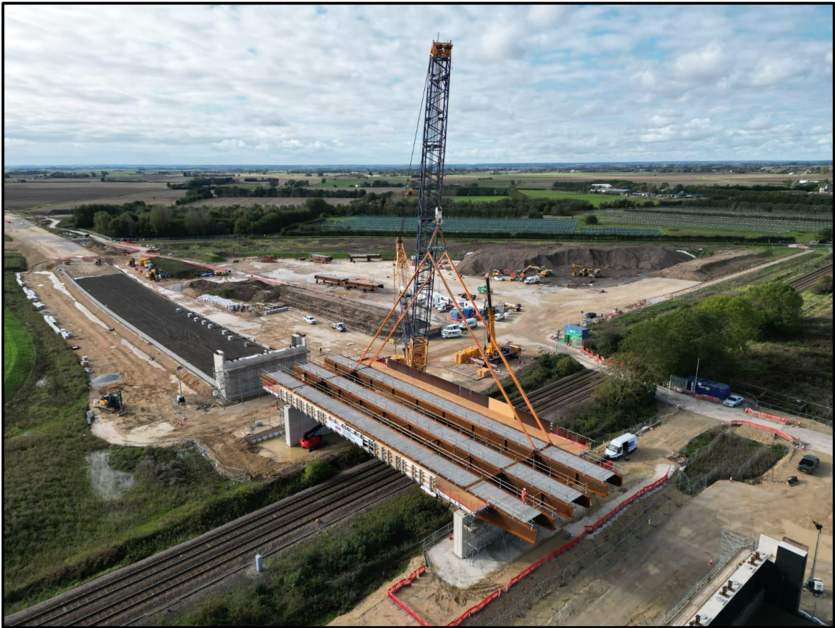
SWRR – All 3 Braced Beams Installed Prior to Rail Track being Opened
