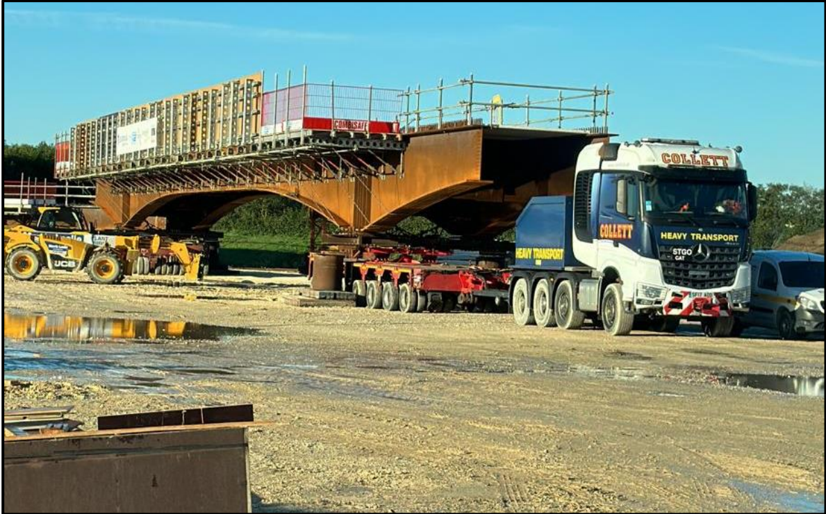
Braced Beams being positioned for installation
