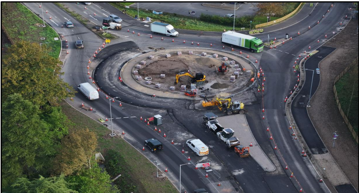
Marsh Lane Roundabout looking North East towards Marsh Lane
