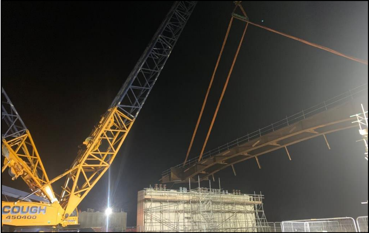
SWRR – Positioning 1 st Braced Beam on Bearings
