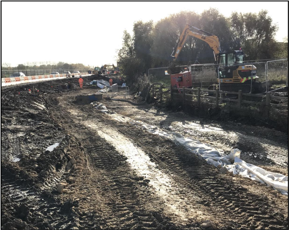
Springfield Road Roundabout South West Quadrant
